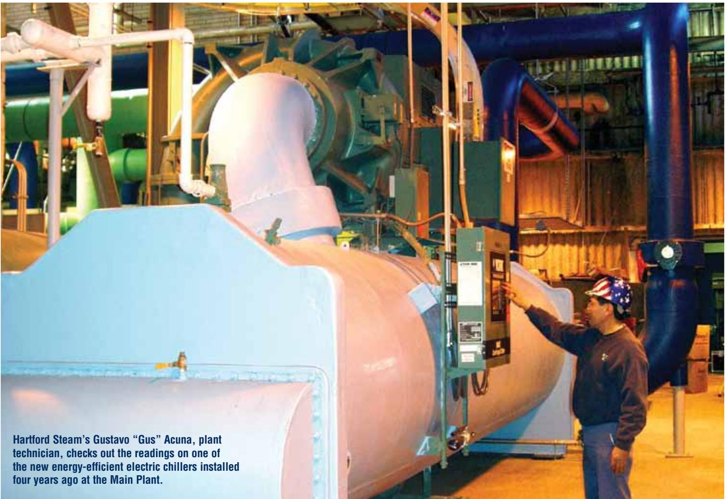
Hartford Steam's Gustavo "Gus" Acuna, plant technician, checks out the readings on one of the new energy-efficient electric chillers installed four years ago at the Main Plant.
