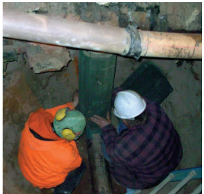
**In March, workers from Hartford Steam's subcontractor D&G Contracting repaired a leaking pipe and added Foamglas® insulation.**
