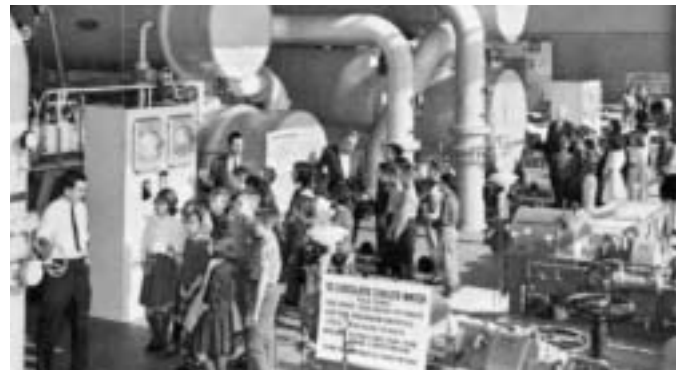
The new plant quickly became a destination for local and international tour groups. This group of fifth graders from Duffy School in West Hartford toured the plant in early 1963. Hartford Steam tour leaders shown here by equipment are John Peak, Al Dudley, Chan Taylor and Fred Pickford.
