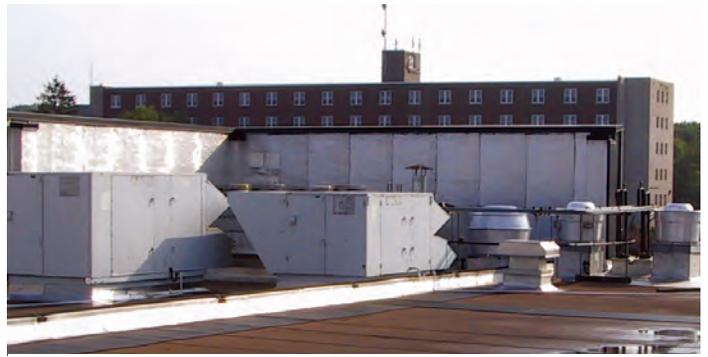
**Exhaust fans are often small but large in number. Other exhaust fans are built into the remote terminal unit. All affect your energy usage.**
